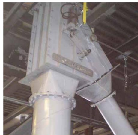
Flap type gravity diverter valve
